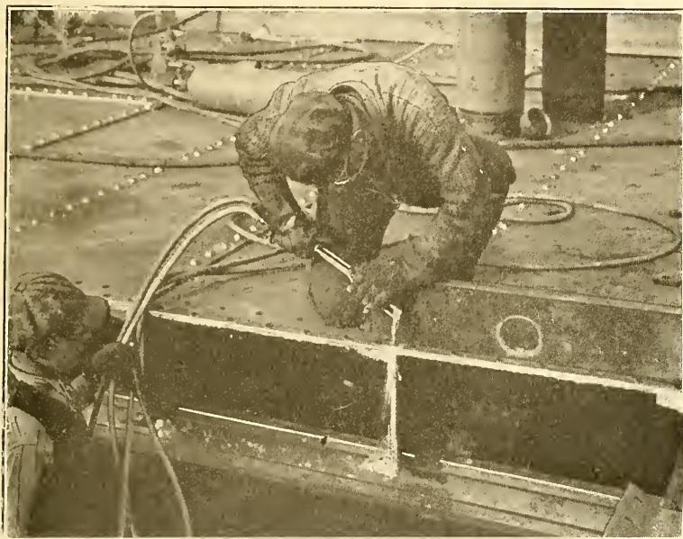
FIG. 222.—Cutting Ship Plates.
